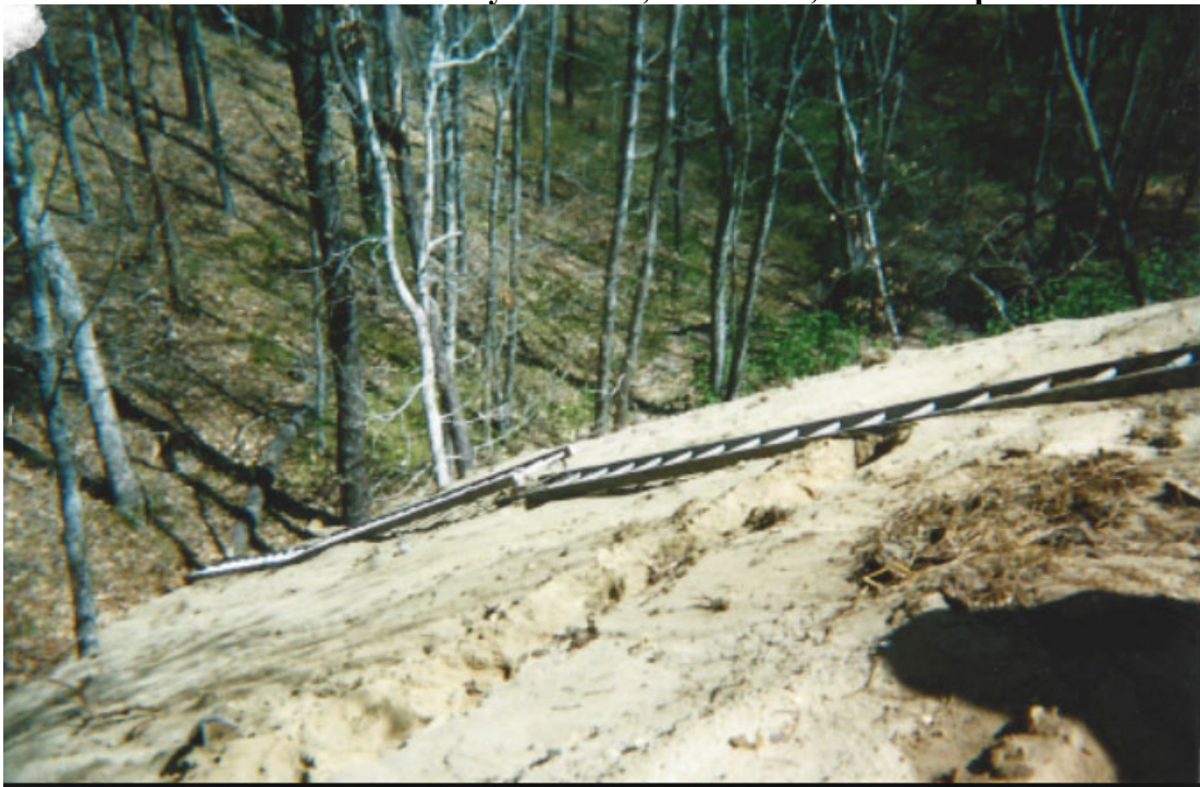
Image by Gordon Peabody. Low impact access and beginning of low profile benching.
