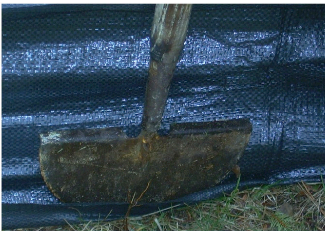
Low tech silt fence installation is effective
