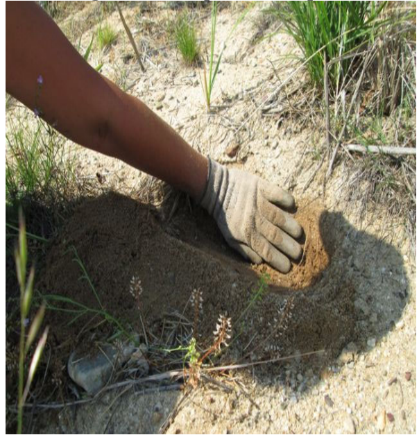
Images by G. Peabody. 24” shelving, using a trowel, forms downslope berm.
