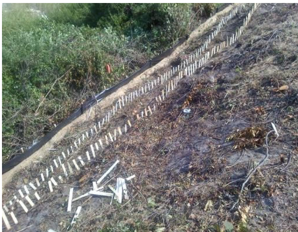
Images by G. Peabody. Limited use of very short fencing helps stabilize site.
