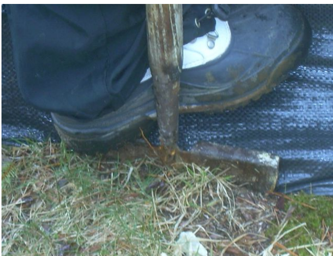
Low tech silt fence installation is effective
