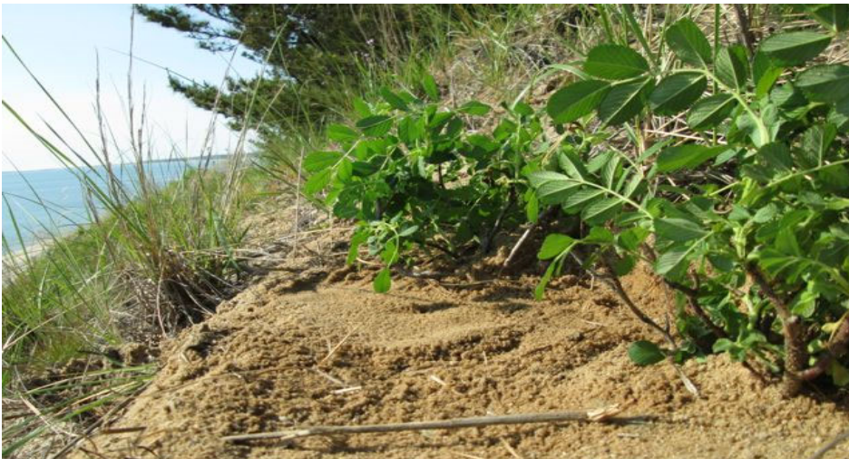
Images by G. Peabody. 24” shelving, using a trowel, forms downslope berm.
