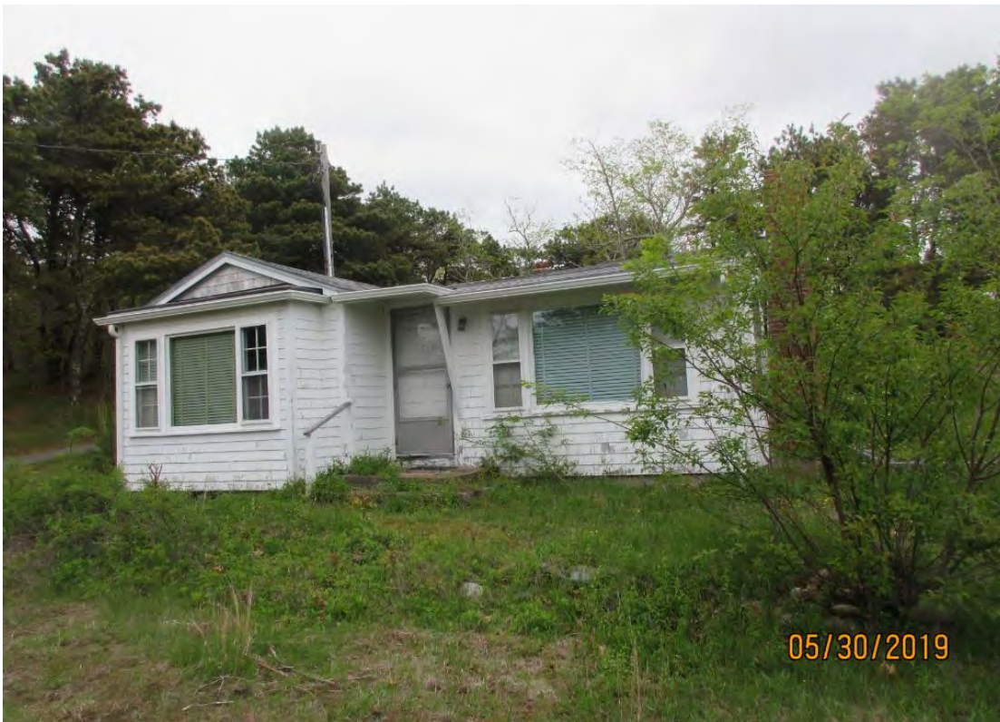
Building # 7 ( with oil heater in basment)
