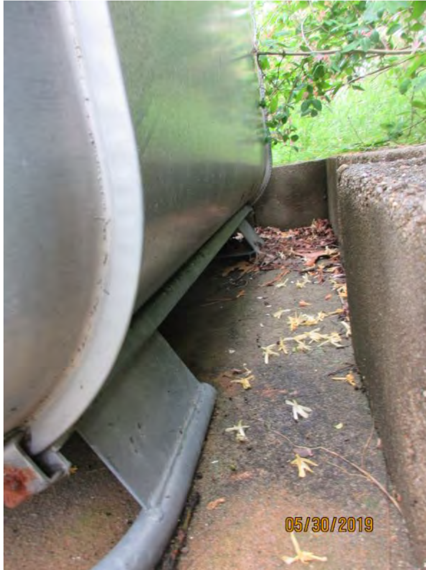
View of AST – no staining
