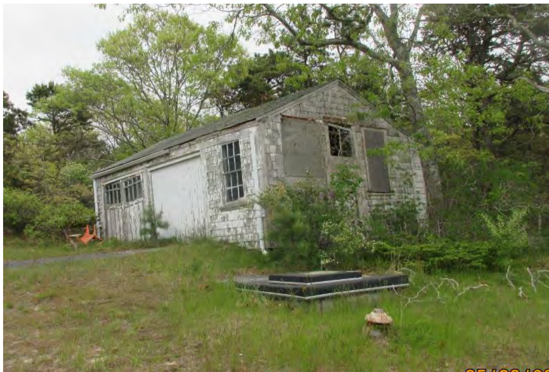
Garage behind building 7C (well frame visible)
