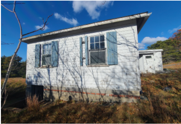
South elevation with access door to crawl space/basement is to the left. Most windows are without storm window protection.
