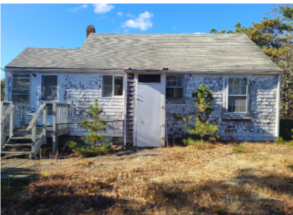
Asphalt shingle roof is past it's useful lief. with small addition above shower stall. Bricks can be seen holding down the edges of the corners of the addition roof.
