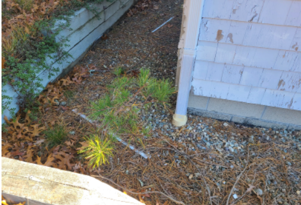
Wood retaining wall set back from building foundation.
