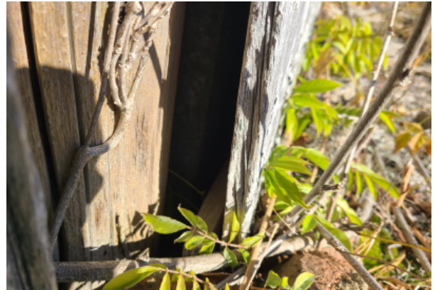
View of foundation pier exposed at one corner.
