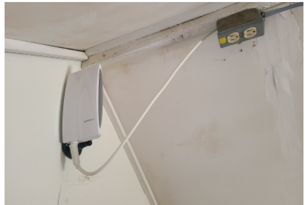
Internet router that is in good condition at roof pitch.
