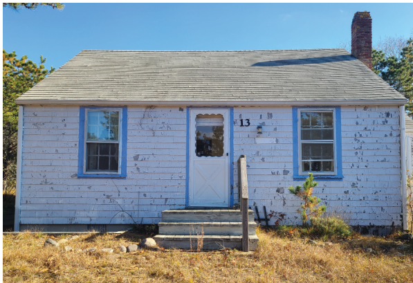
Front elevation of the building, concrete steps with insufficient railing, and original windows that need replacing.
