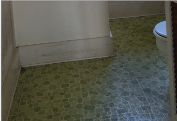
Vinyl sheet tile in bathroom with with painted wooden base showings.
