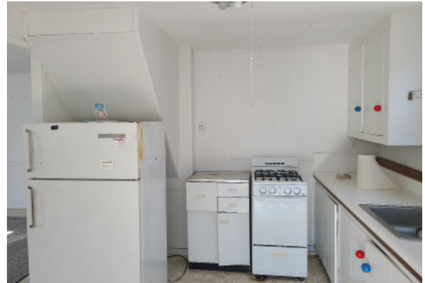
Kitchen with refrigerator, stove/oven, and in counter sink. Both the stove/oven and refrigerator are outdated and need replacing.
