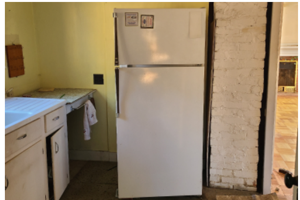
Refrigerator that is outdated and needs replacing. Beside it can be seen what seems to be an old chimney that has been abandoned.
