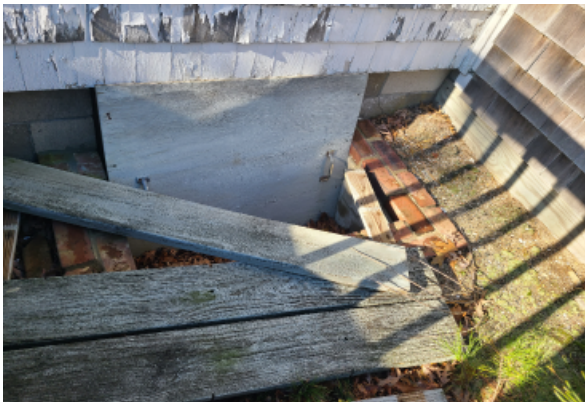
Access panel to crawl space
