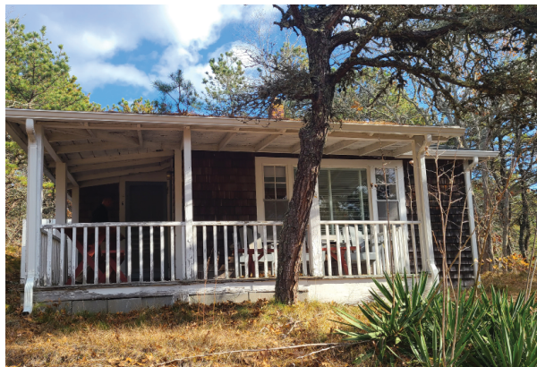
View of the front of the building, with a covered porch addition, and addition to the left side. The grade at this location slopes North (left) to South (right).
