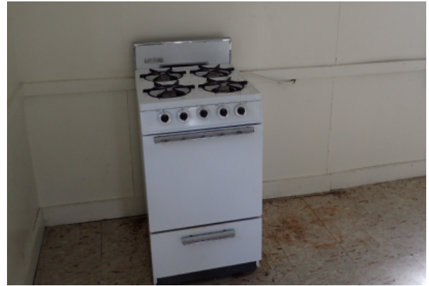
Stove/oven fixture with exposed connection into the wall. Fixture is outdated and needs replacing.
