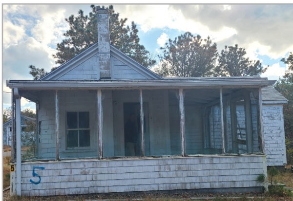
Front of cottage where a covered porch wraps around one corner. The screens and low walls are greatly weathered.
