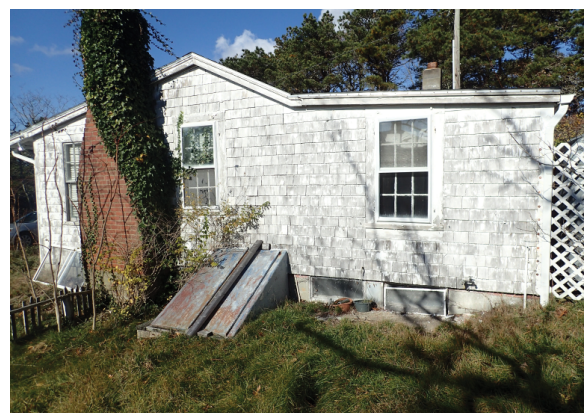
South elevation, vegetation penetration can be seen.
