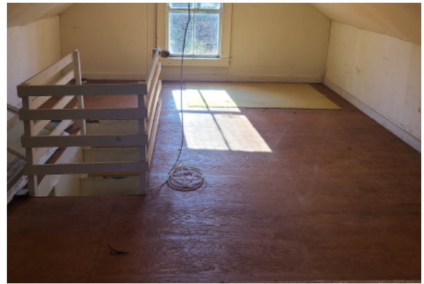
Second level flooring is exposed wood boards.
