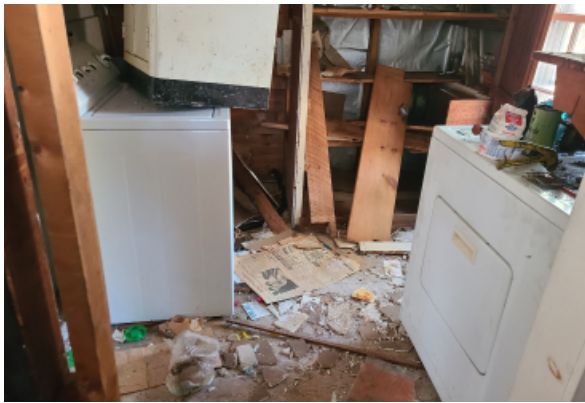
A set of clothes washer and dryer, as well as another unidentified fixture on top. The condition of these fixtures are unknown, but any utility connection must be updated.
