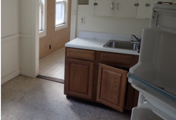
Refrigerator and in counter double sink are present. The refrigerator has signs of mold, and must be replaced.
