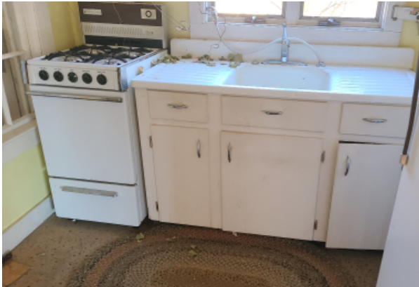
Stove/oven fixture with counter top sink fixture. The hardware on the sink is non-compliant, and the stove/oven fixture is outdated and needs replacement.
