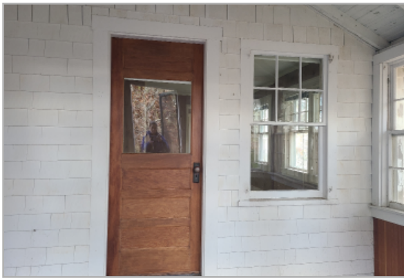
View from front porch additon to main entrance.
