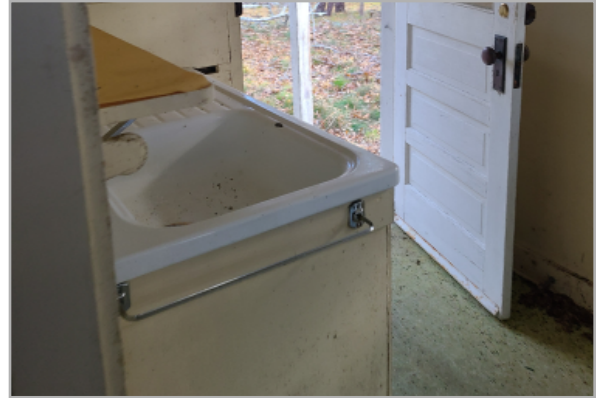
Porcelain sink and counter unit in kitchen. The green linoleum flooring has tested positive for asbestos.
