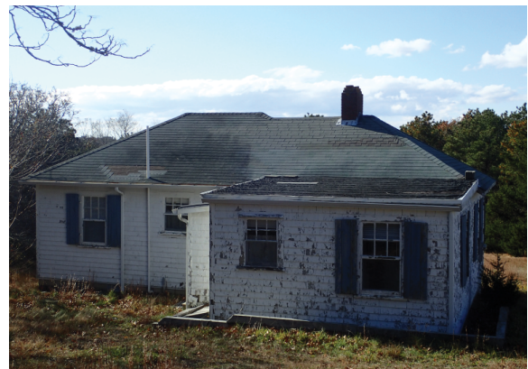
The cottage has gutters at every eave, but some downspouts are missing, and all aluminum is failing.
