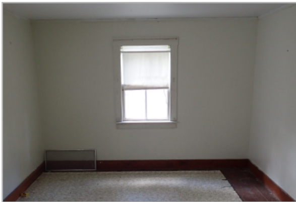
View of painted interior wall with base trim, there are areas of mildew growth on the wall panels.
