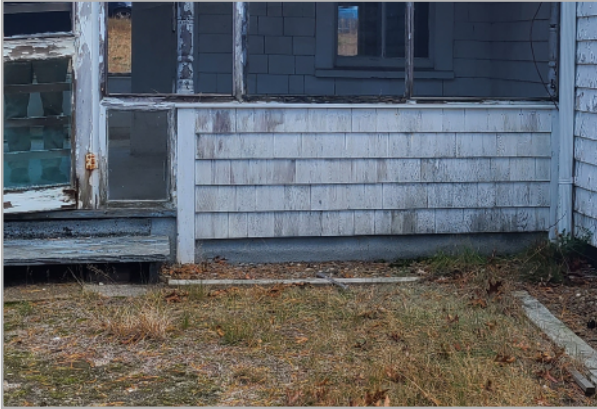
Wooden foundation under front porch addition sitting on grade.
