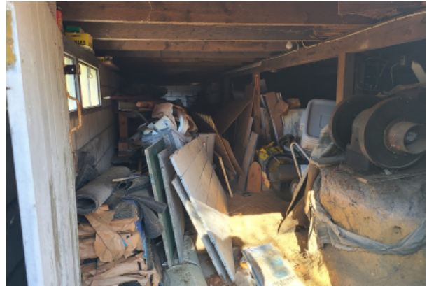
View inside crawl space/basement.
