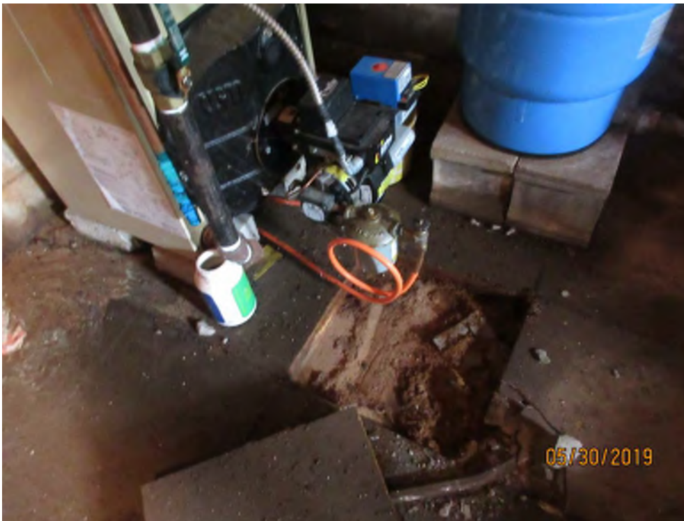
View of oil burner in basement of number seven. Floor tile removed to collect soil sample.
