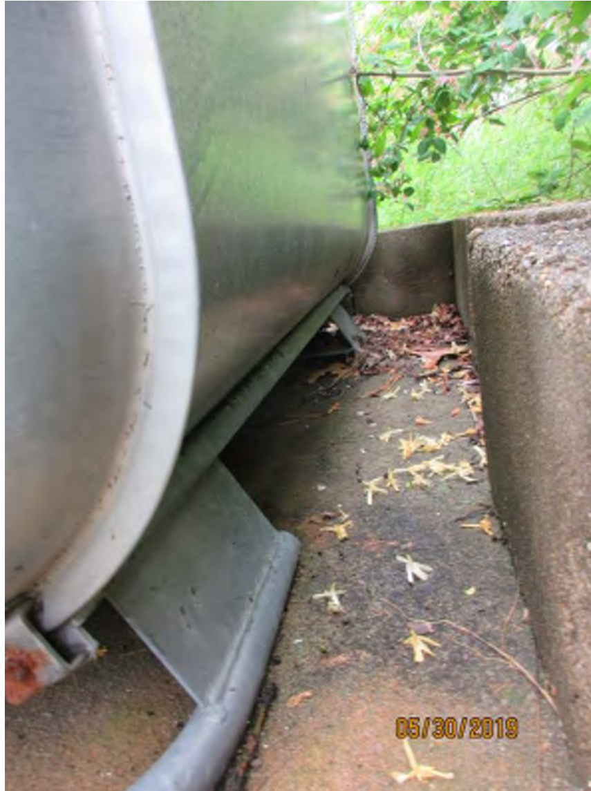
View of AST – no staining
