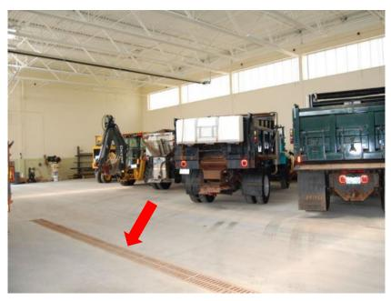
Any drips or spills from vehicles stored inside will be collected in a closed floor drain system preventing them from reaching the environment
