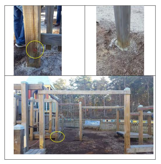
Repaint the painted depth markings to facilitate future maintenance. If necessary, measure up 12" from the bottom of the EWF to locate new stripes. Add engineered wood fiber until the compacted depth is 12" throughout.
