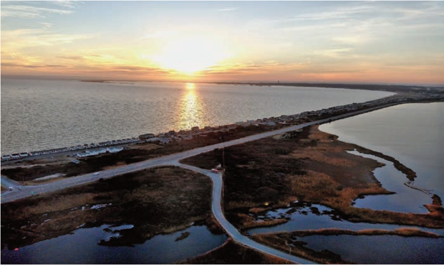
East Harbor at Sunset prior to Culvert repair completion.. Photo Courtesy of Jeffrey Souza
