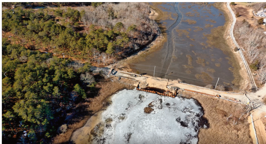
Eagle Neck Creek culvert project. Photo Courtesy of Jeffrey Souza
