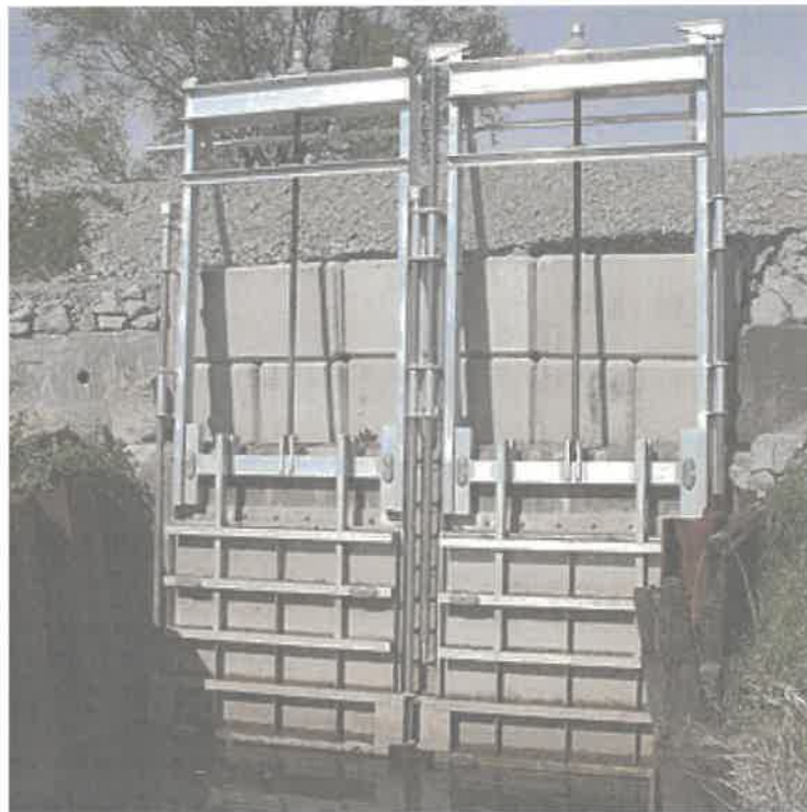
Figure 7. Golden Harvest GH-50 sluice-flap combination gate.
