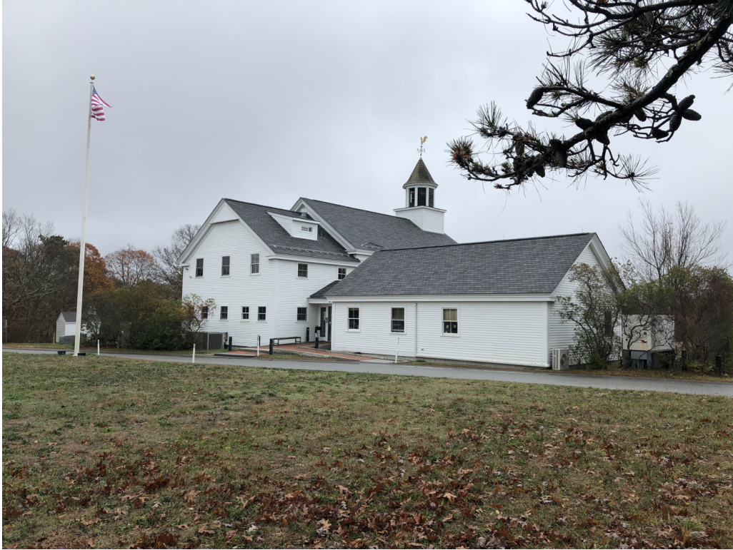
Photo 1: View looking southeast at the Town Hall.
