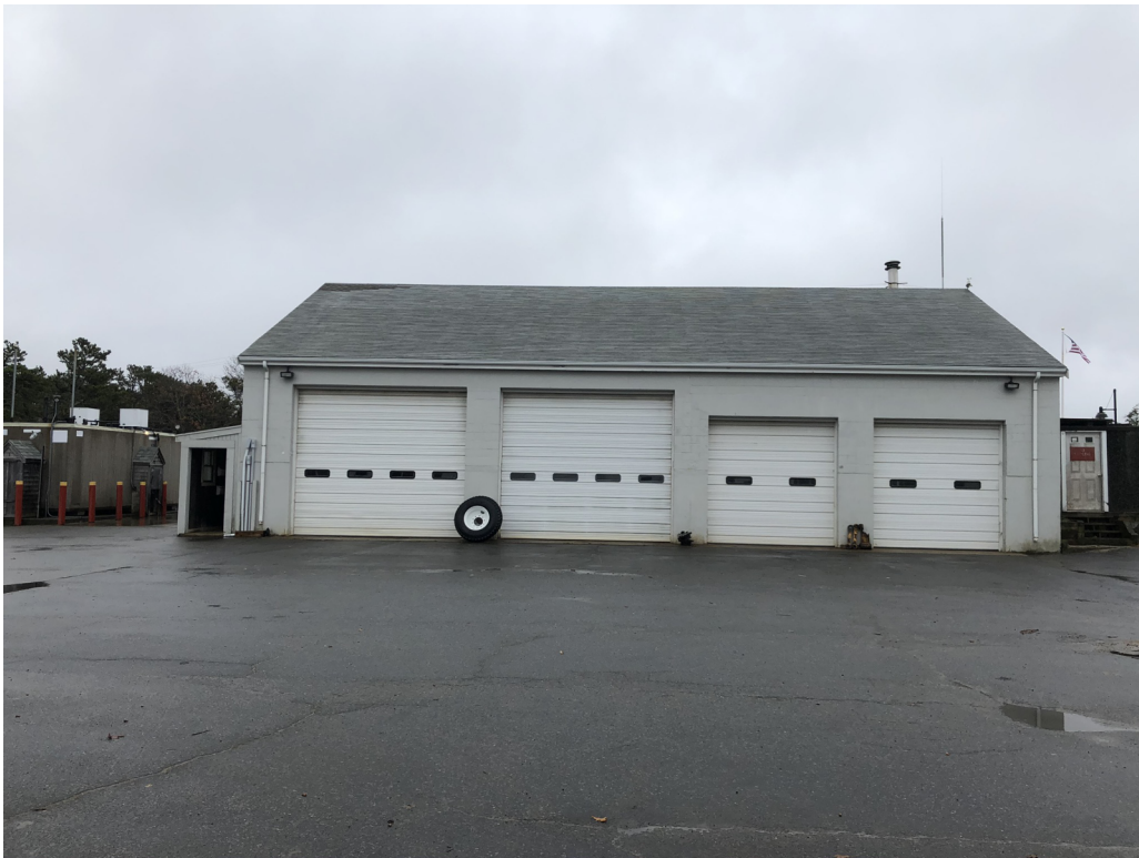
Photo 2: View looking southwest at the main garage and fueling station.
