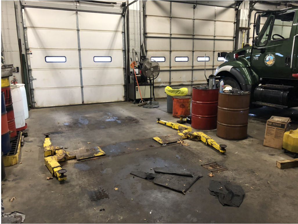
Photo 15: View looking north at subgrade hydraulic lift in main garage.
