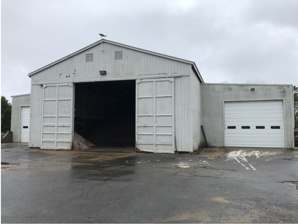
Photo 3: View looking west at the salt/sand storage shed.
