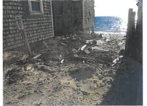
BETWEEN BLDG. 2 & BLDG. 3 12-27-2022
