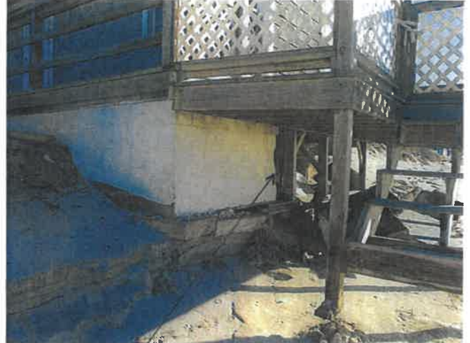
NOTE: EMERGENCY SHORING IN PLACE
