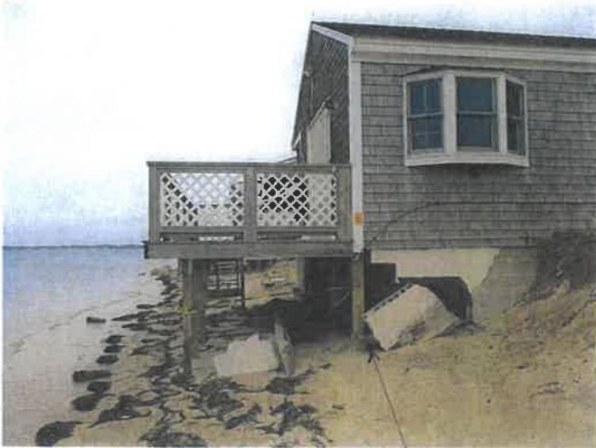
NOTE: EMERGENCY SHORING IN PLACE
