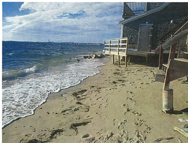
BUILDING 3 LOOKING WEST - NOTE HOW CLOSE TIDE IS TO BUILDING
