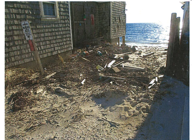
BETWEEN BLDG. 2 & BLDG. 3 12-27-2022
