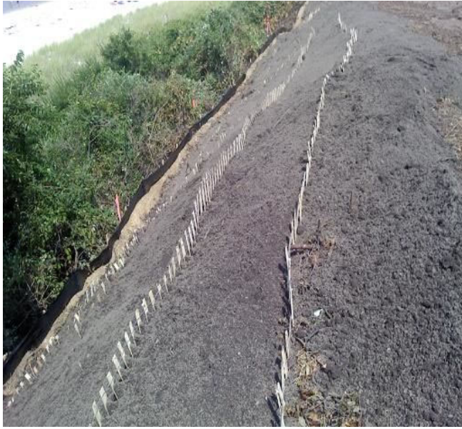
Images by G. Peabody. Stages in the bioengineered, slope stabilization process.
