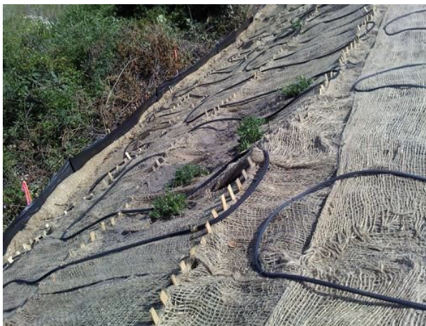
Images by G. Peabody. On this site we planted woody stems through netting.
