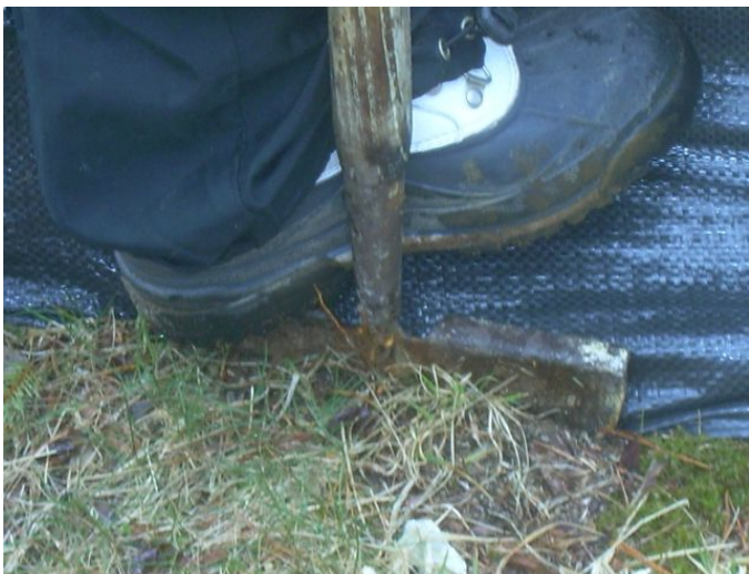
Low tech silt fence installation is effective
