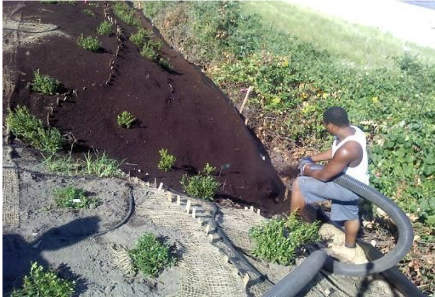
Image by G. Peabody. Blowing in mulch significantly reduces site impacts.
