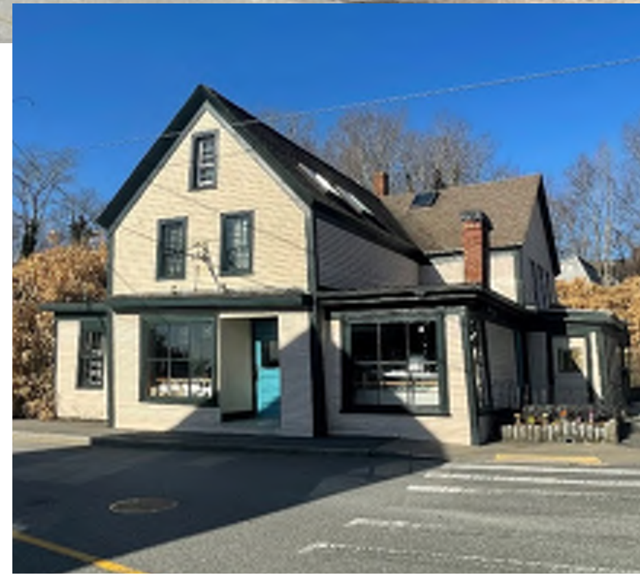
Figure 13: Small-Scale Commercial Buildings Examples
