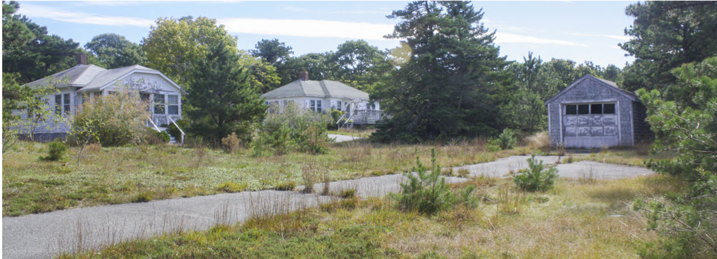
There are eight uninhabited wood frame cottages currently on the Walsh Property, which is accessed via Walsh Way.
