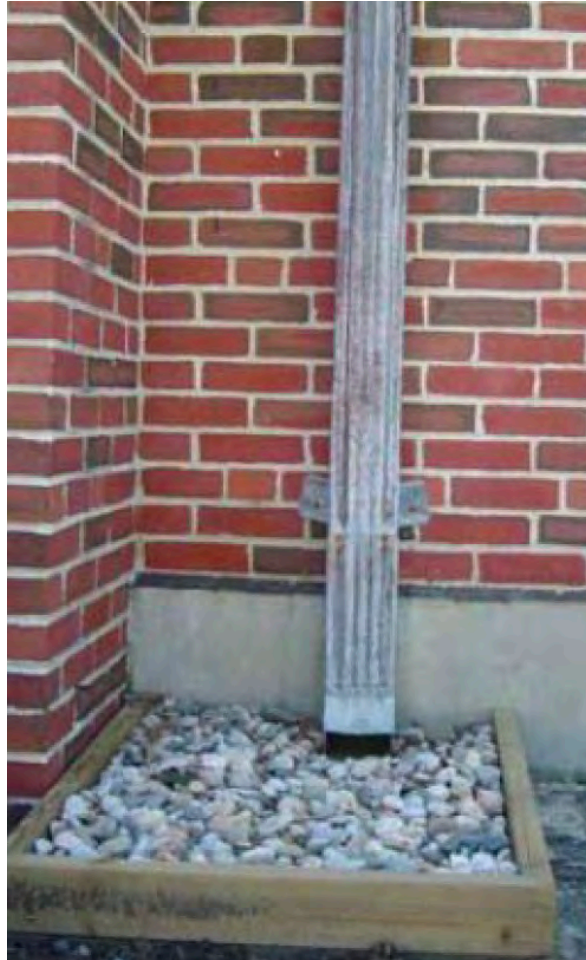
Infiltration of Roof Runoff
