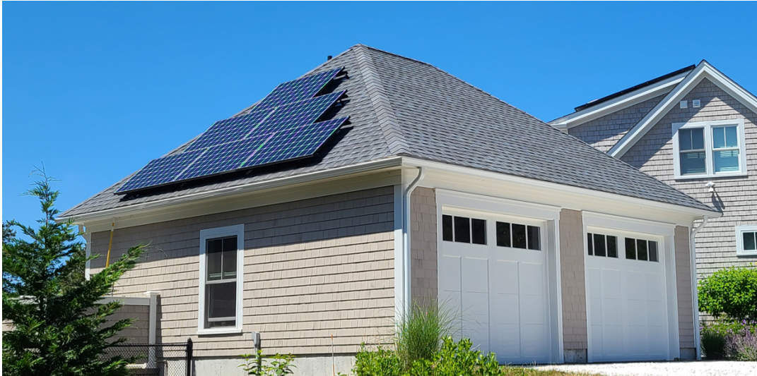
Hip Roof with Solar
