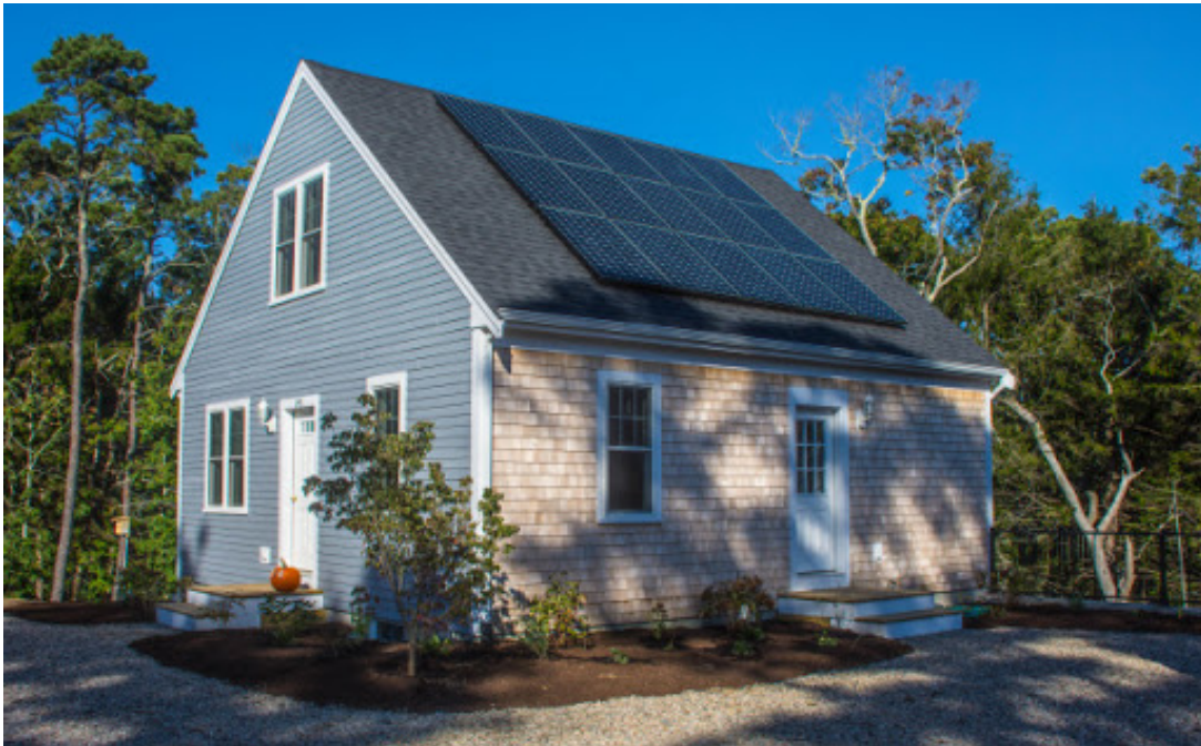
Gable Roof with Solar
