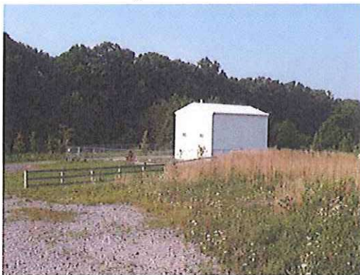
Wastewater treatment plant building
