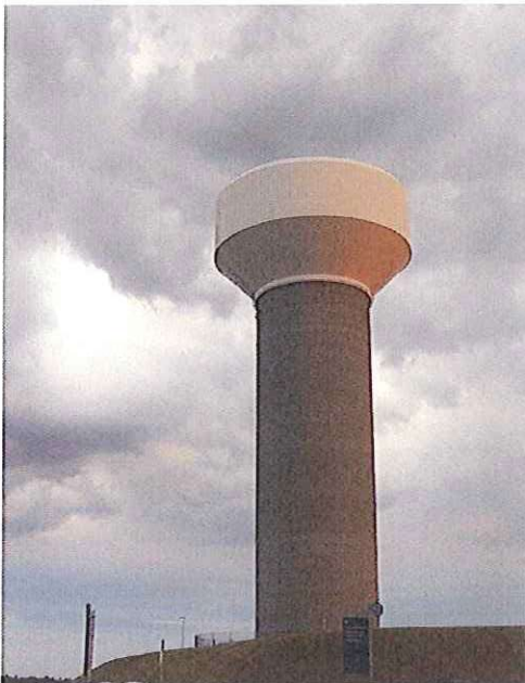
Elevated 1900 m 3 (500 000 gal) water storage tank for reclaimed water at Gillette Stadium.
