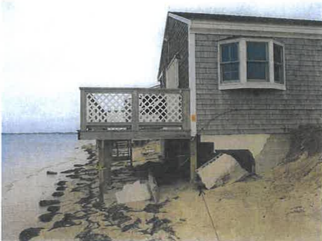
NOTE: EMERGENCY SHORING IN PLACE
