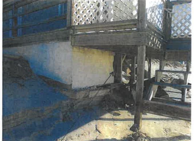
NOTE: EMERGENCY SHORING IN PLACE
