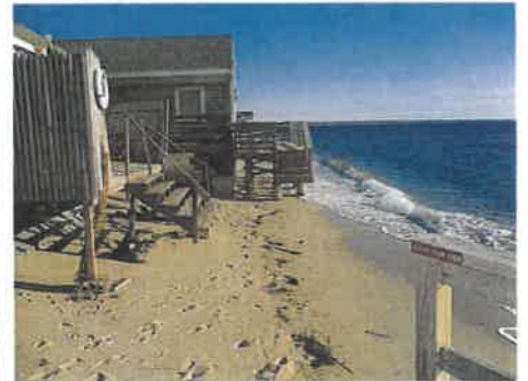
BUILDING 1 - LOOKING EAST
