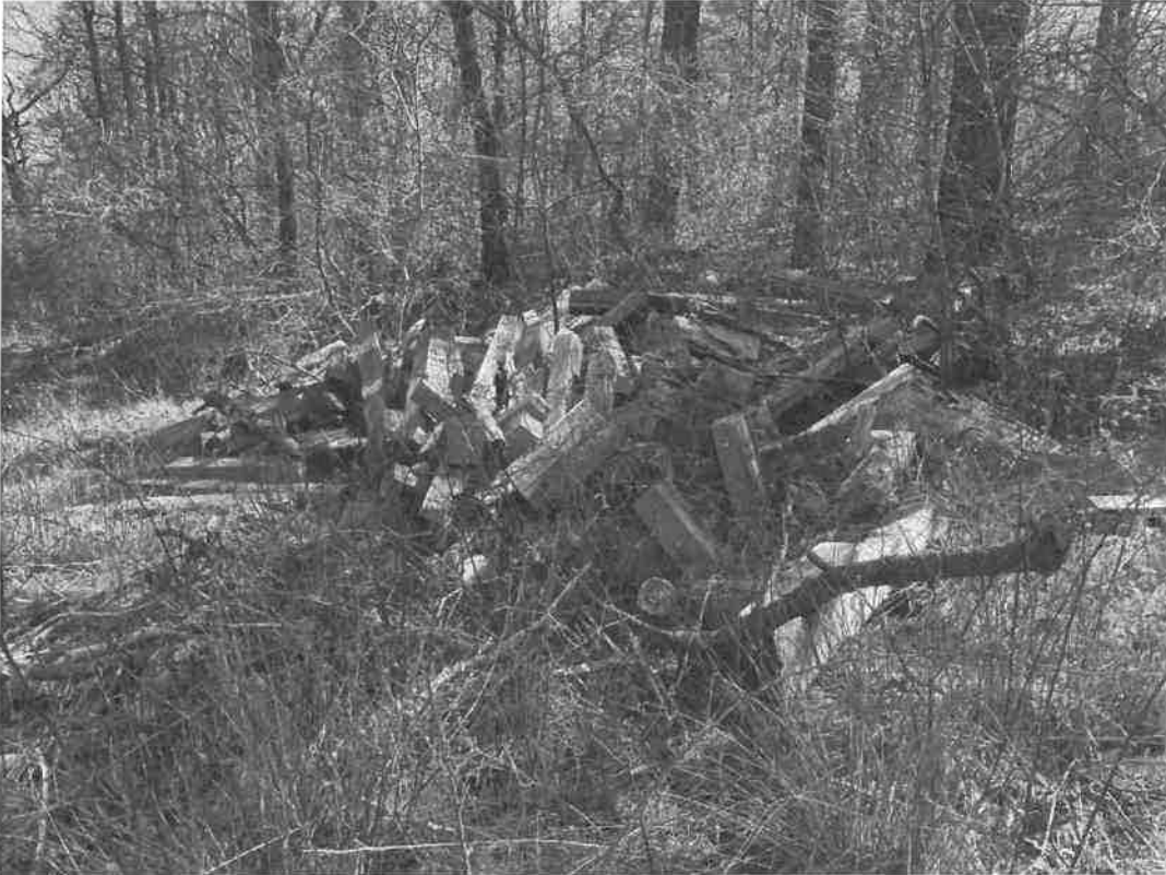
Photograph #5—View of a debris pile consisting of timber located within the northern portion of the site. The debris within and near the work area is proposed to be removed.
