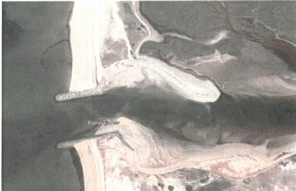
Pamet Harbor 2010 (after work on the groin and the dune/beach)
