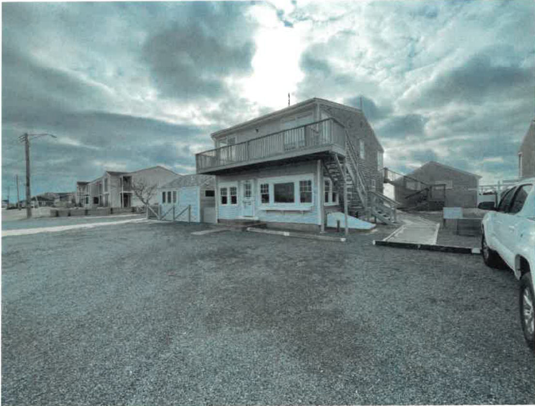
Photograph #1 – View south from Shore Road of the existing structures onsite.
