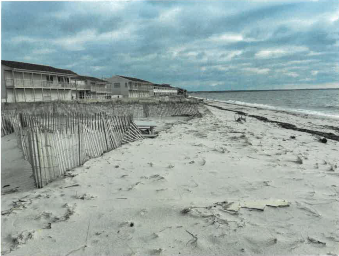
Photograph #5 – View east across the southern portion of the site near the Dune/Beach boundary. Recent storm damage has eroded the Dune face at the site.
