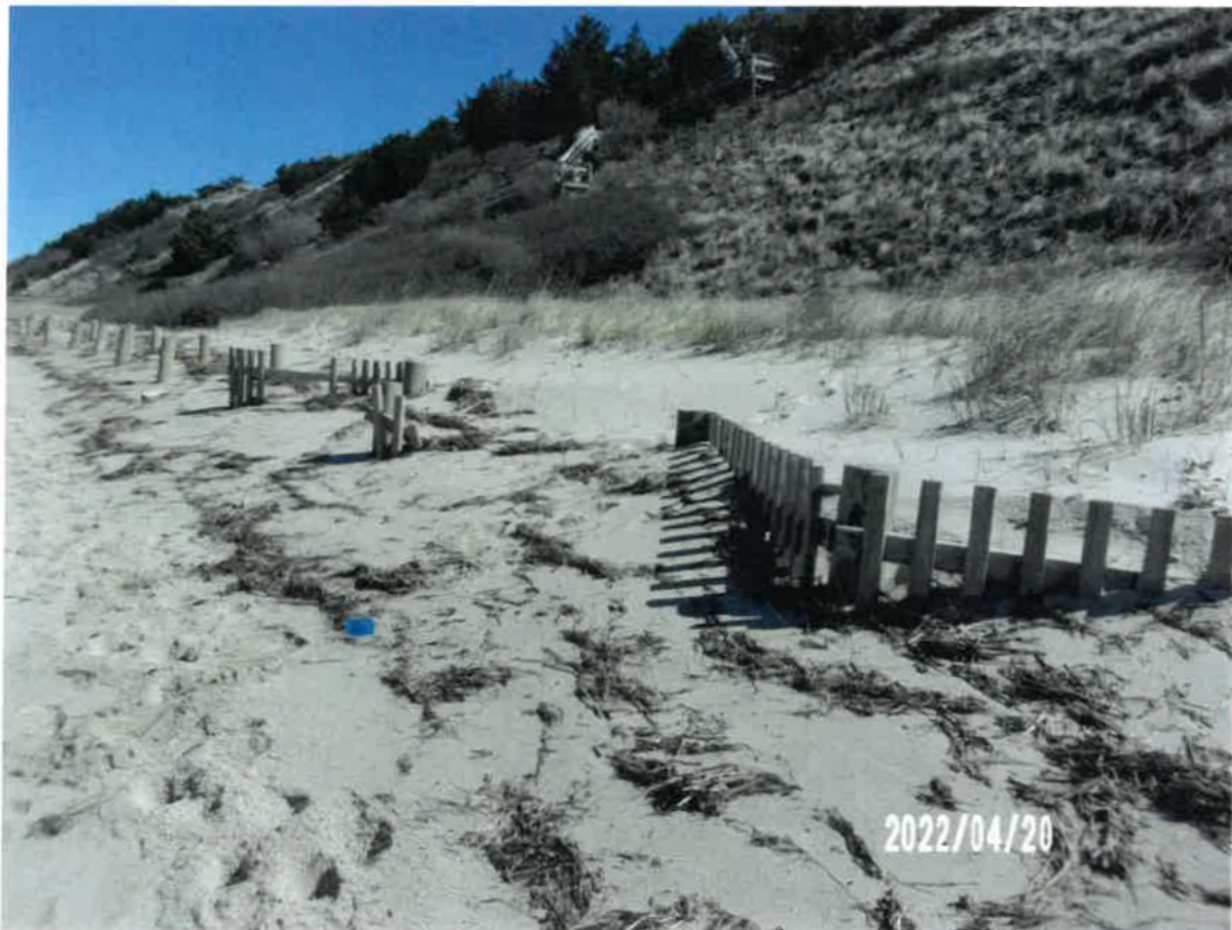
Photograph #2 - View north along the existing sand drift fence. Many existing support piles will need to be raised and resecured.
