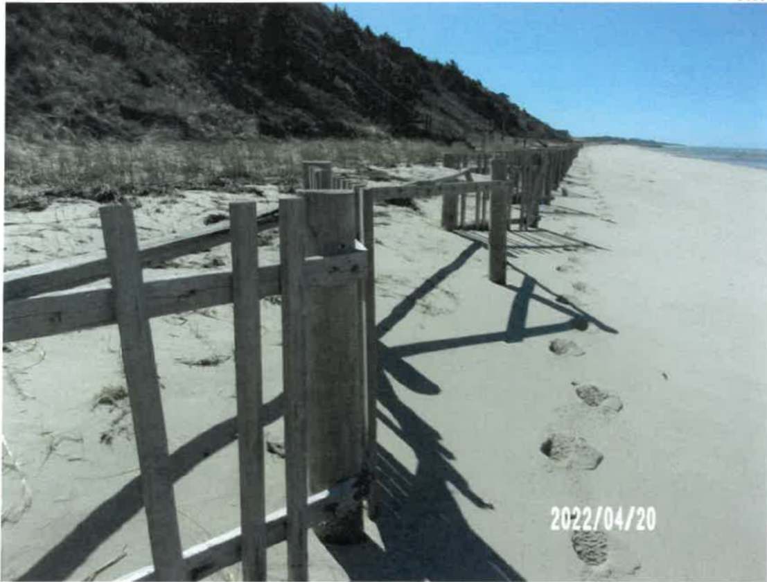
Photograph #1 – View south along the existing sand drift fence.
