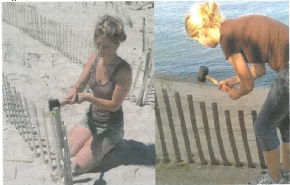
Safe Harbor images by Gordon Peabody. Installation of 24" sand fence
