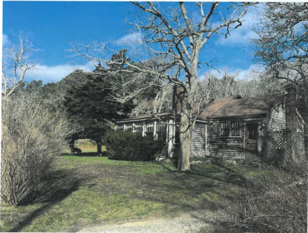
Photo 2 Longnook Road (South) Elevation
