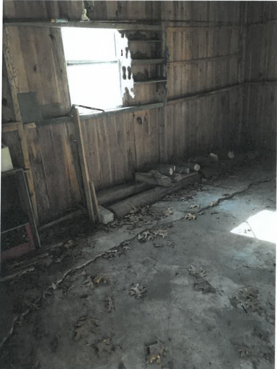
Photo 13 Garage Floor and Wall Framing
