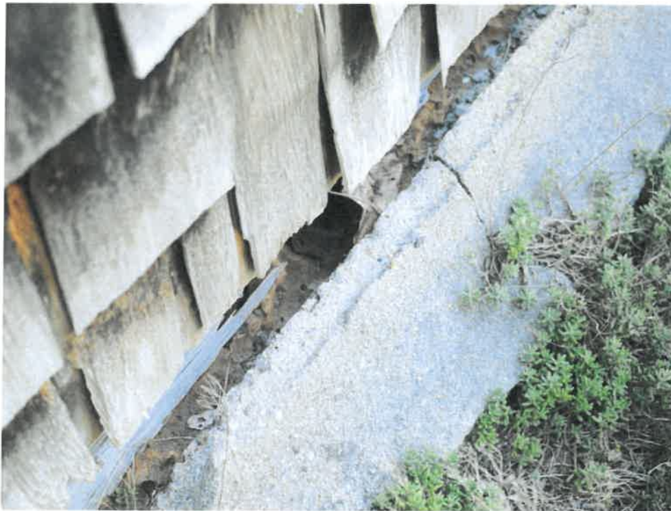
Photo 10 House West Elevation @ Critter Entry Point and Foundation Repair
