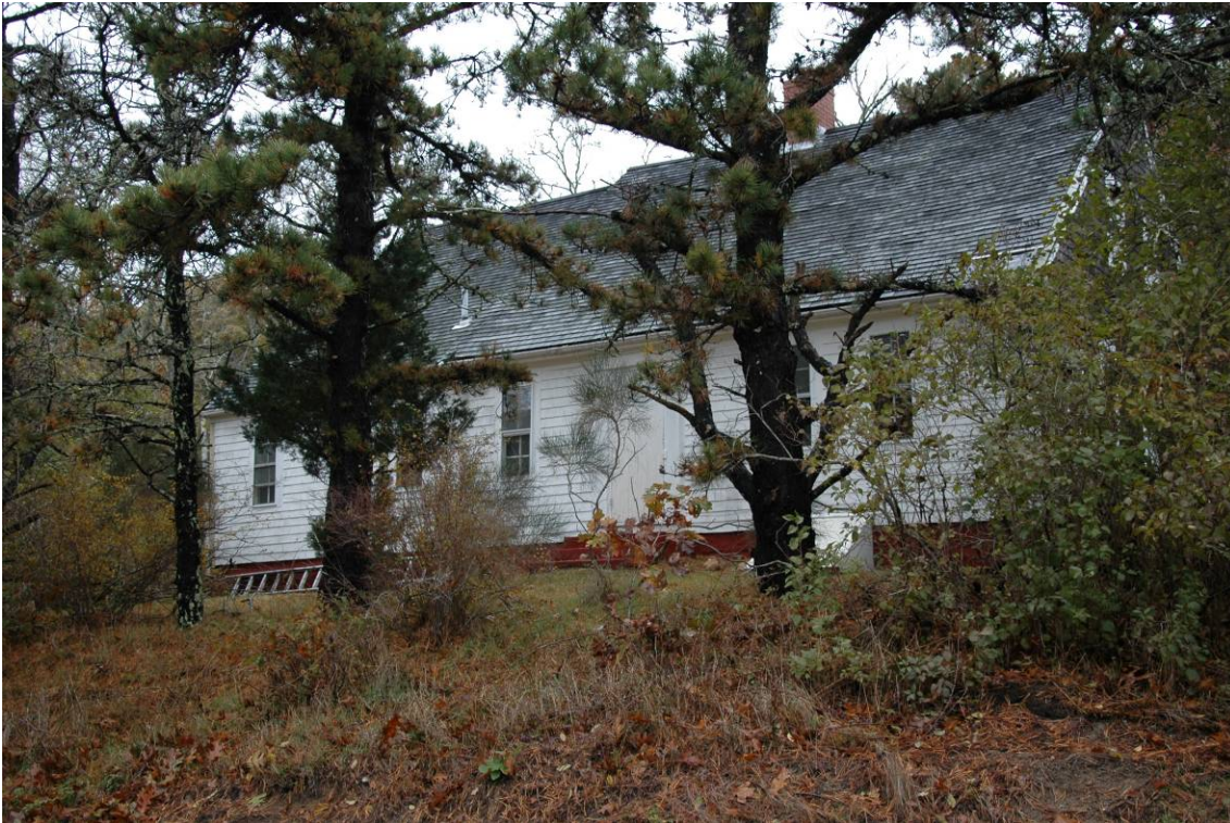
Photograph 1. View looking northwest toward house from North Pamet Road.
