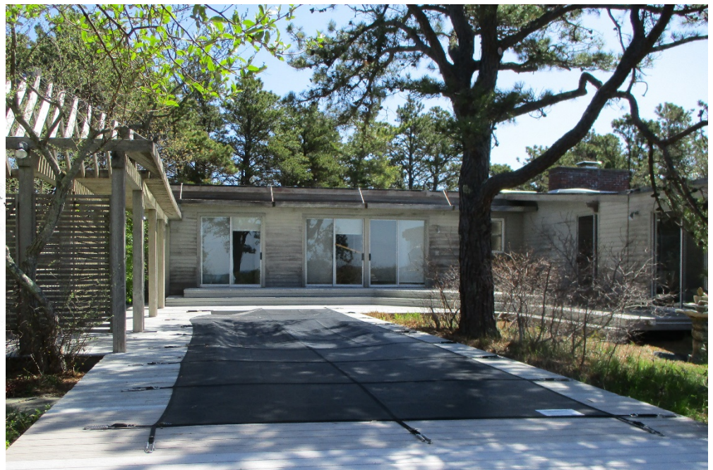
Photo 2. View of rear elevation, looking east (2019 Assessor).
