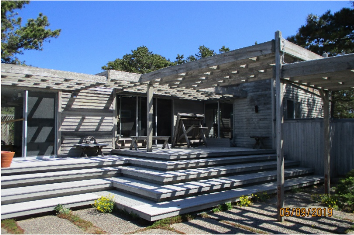
Photo 3. View of S elevation (partial), looking NE (2019 Assessor).
