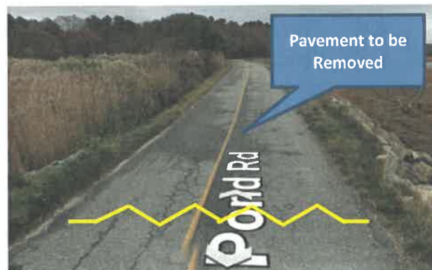
Figure 13 — Approximate Limit of Pavement Removal and Channel Breach South of Mill Pond Culvert (facing south)
