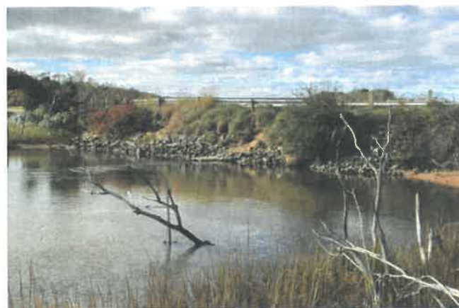
Figure 5 — Upstream Culvert Outlet and Stone Armor Slope Protection (facing south)
