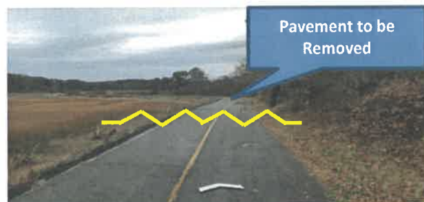
Figure 12 — Limit of Pavement Removal South of Mill Pond Road / Post Drive Intersection (facing north)
