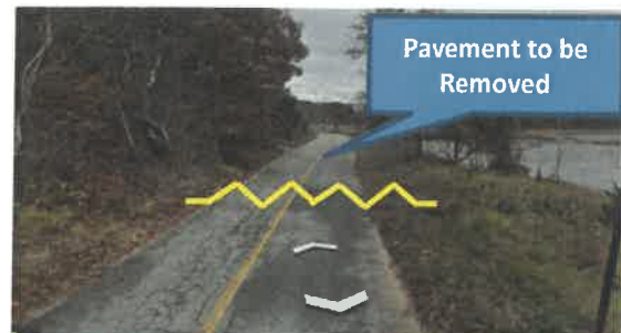
Figure 10 — Limit of Pavement Removal South of Mill Pond Road / Depot Road Intersection (facing south)
