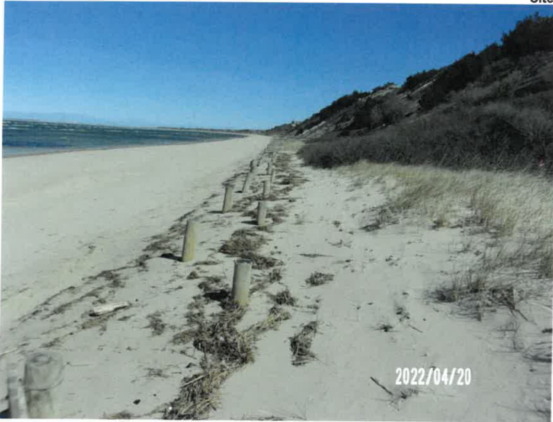
Photograph #3 – Another view north along the existing sand drift fence where much of the fencing sections will need to be replaced.
