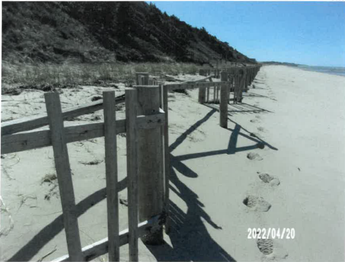
Photograph #1 – View south along the existing sand drift fence.
