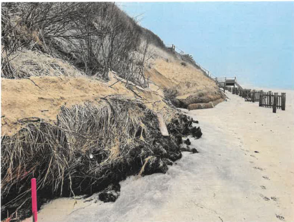
Photograph #2 - View looking southeast along the toe of the bank onsite.
