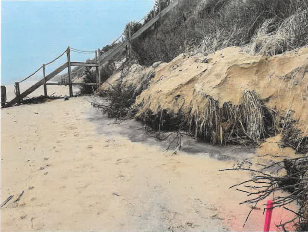
Photograph #1 – View looking northwest along the toe of the bank onsite.
