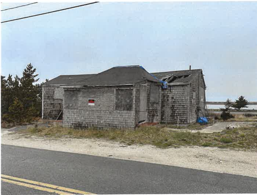
View from Shore Rd.
