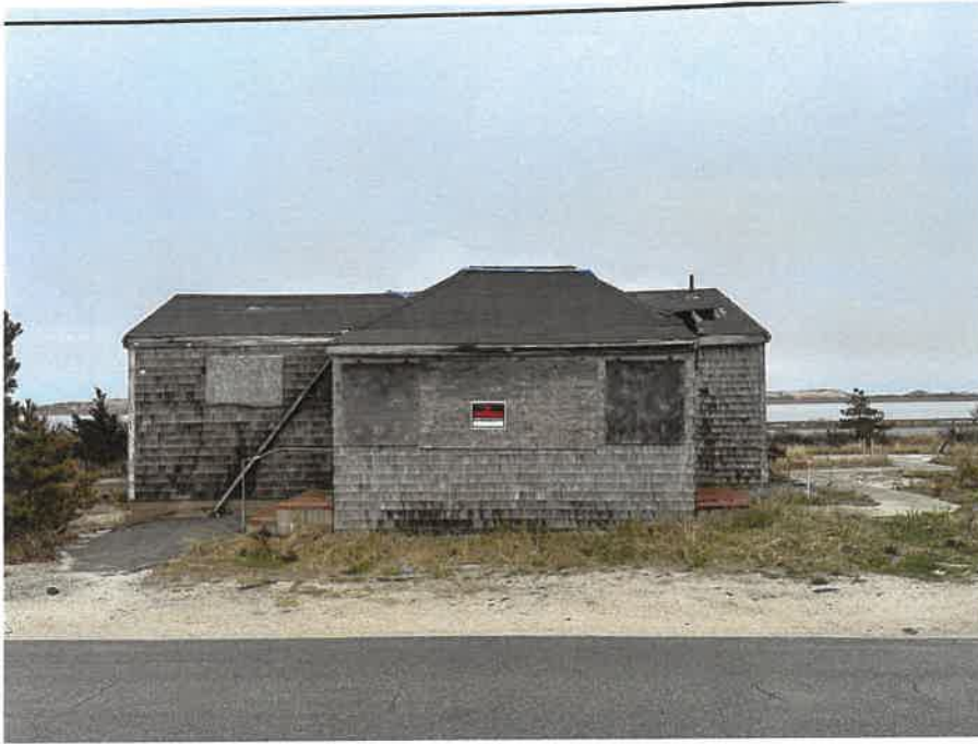
View from Shore Rd.
