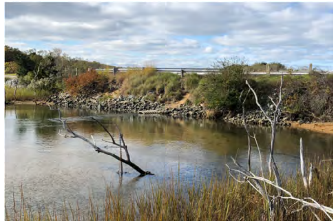
Figure 4 — Upstream Culvert Outlet and Stone Armor Slope Protection (facing south)
