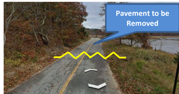
Figure 9 — Limit of Pavement Removal South of Mill Pond Road / Depot Road Intersection (facing south)
