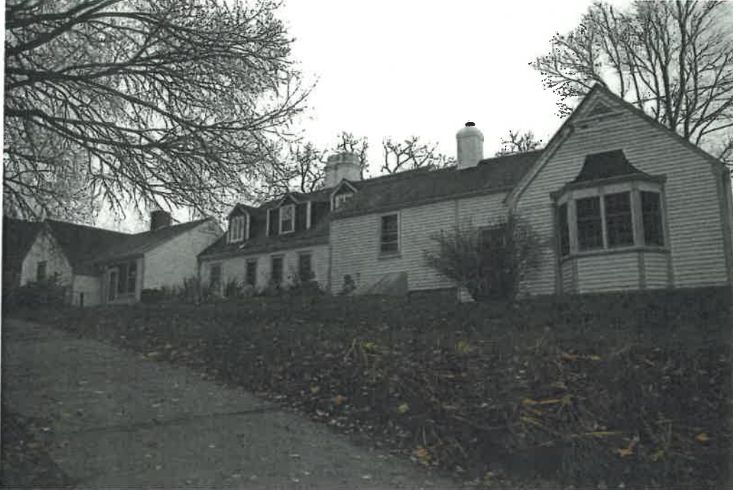
Photograph 1. View looking southeast toward house from road.
