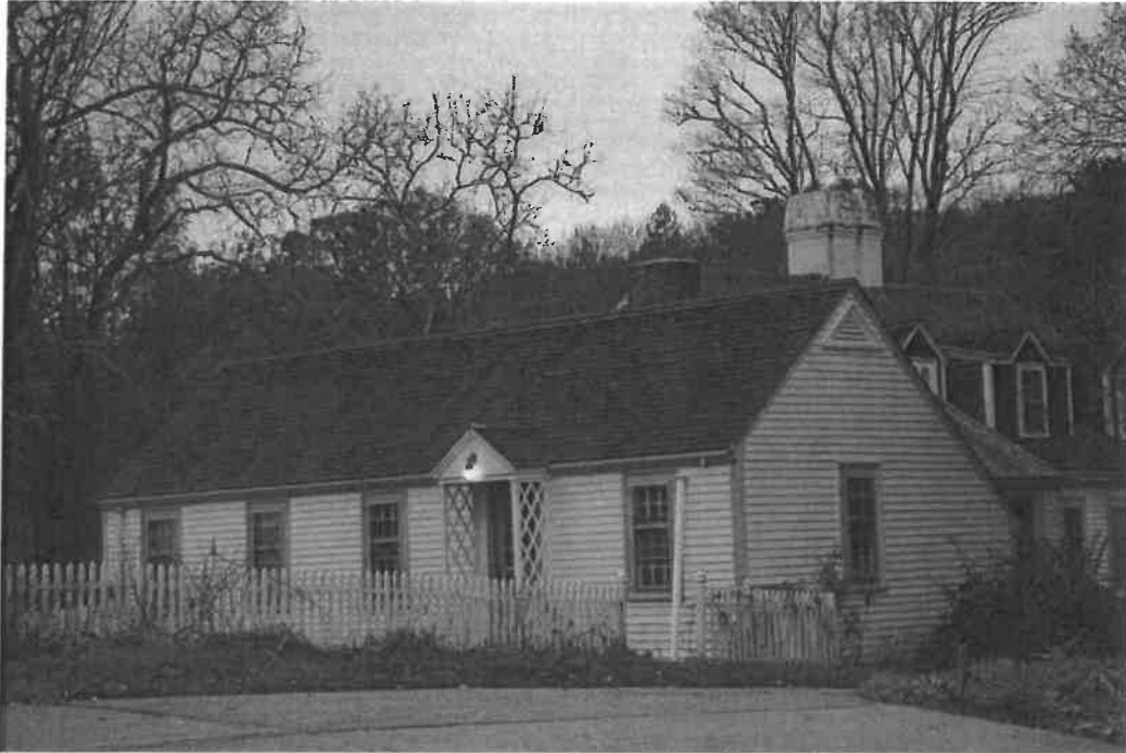
Photograph 3. View looking southwest toward east ell from driveway.
