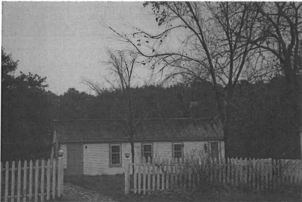
Photograph 4. View looking south toward cottage from parking lot.
