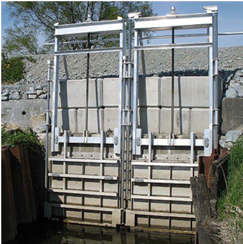
Figure 1. Example of a Golden Harvest GH-50 sluice-flap combination gate.
