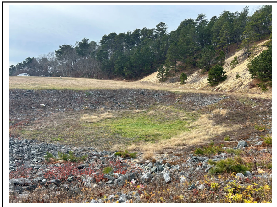
Photo 2: Landfill stormwater detention basin.
