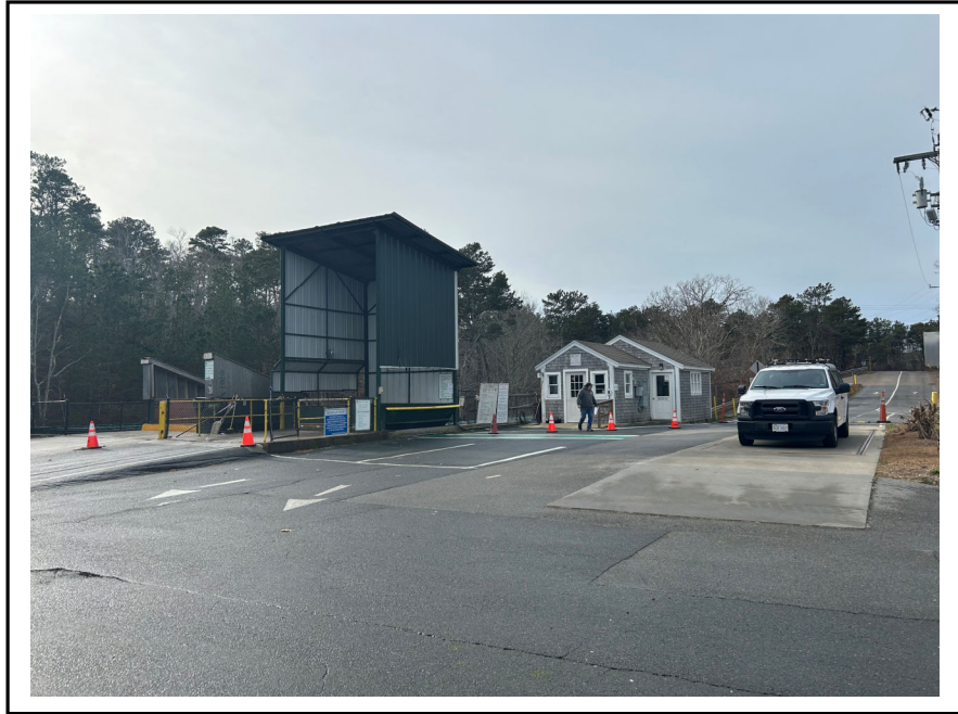
Photo 3: Site entrance, scale and scale house.
