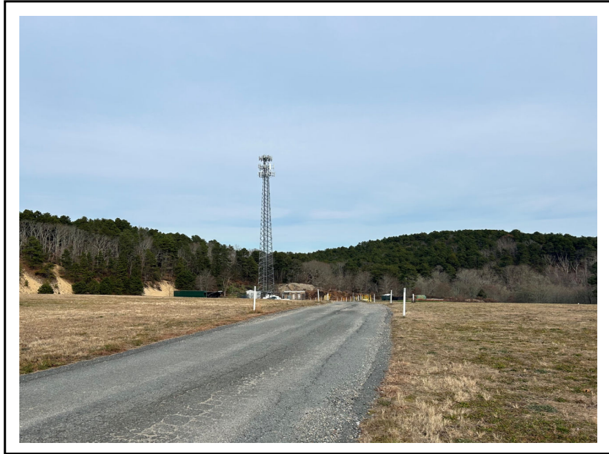
Photo 3: Landfill access road and stable landfill cover.
