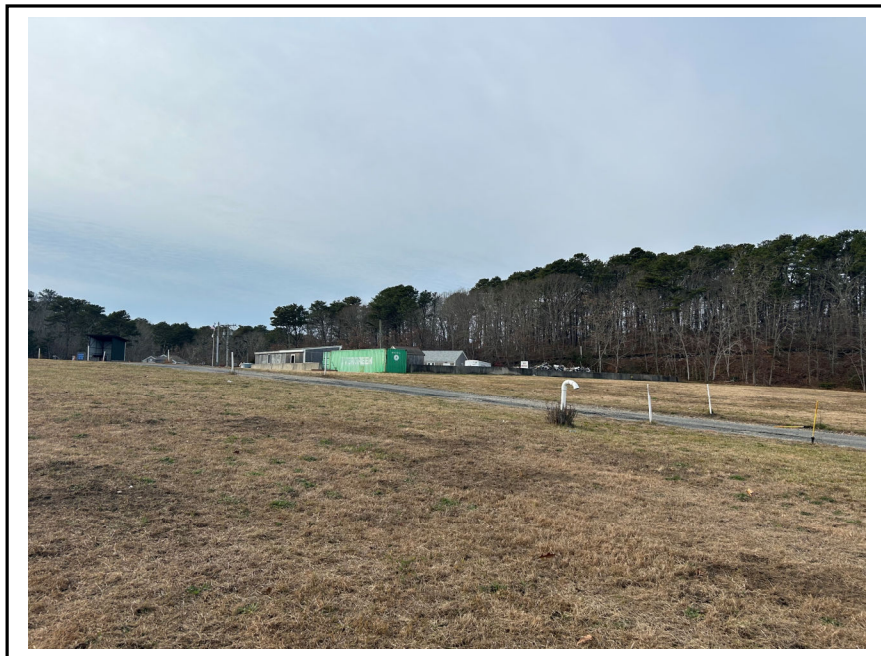
Photo 6: Landfill transition to transfer station area.
