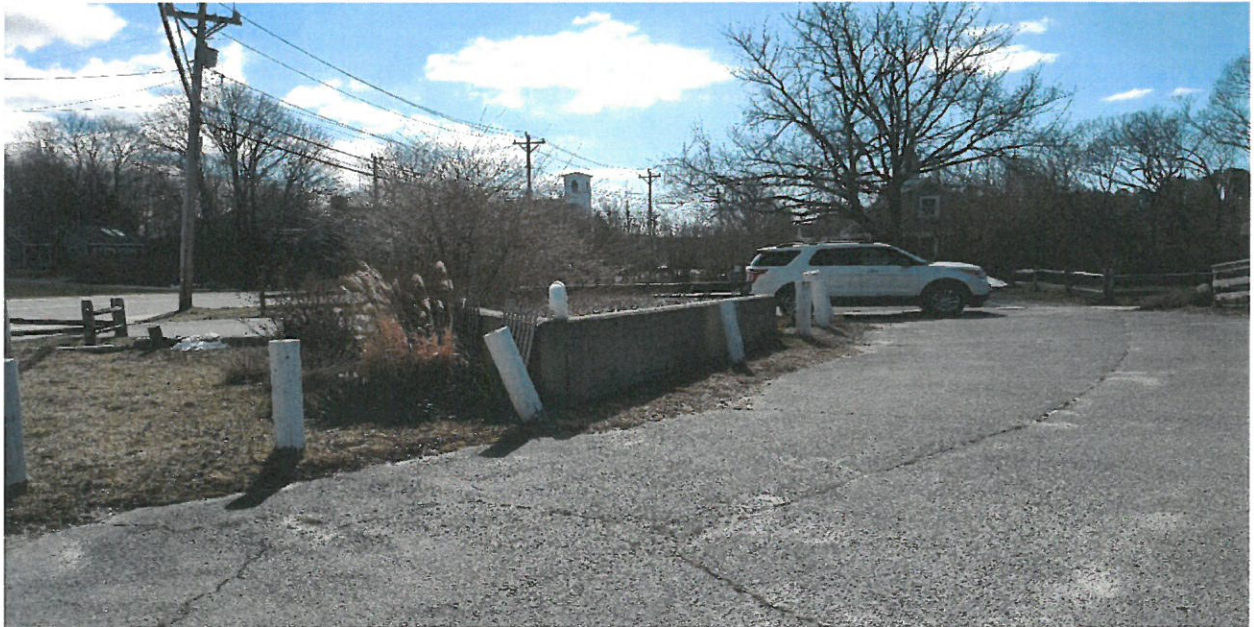
38 Shore Rd- raised concrete containment wall for leach field
