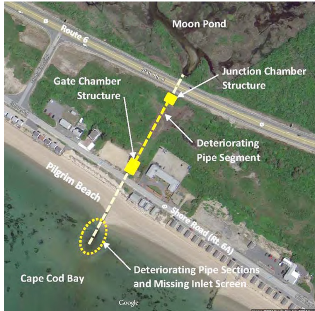
Figure 4.6 | Aerial image of the deteriorating and vulnerable characteristics of East Harbor Culvert. From the Final Report: East Harbor Culvert Evaluation (Woods Hole Group, 2015)
