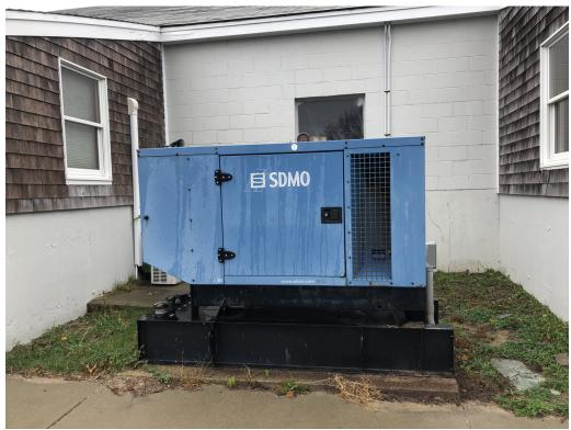
Photo 14: View looking north at the main garage emergency diesel generator.
