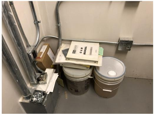
Photo 9: 5-gallon buckets of hydraulic oil adjacent to elevator pump motor.
