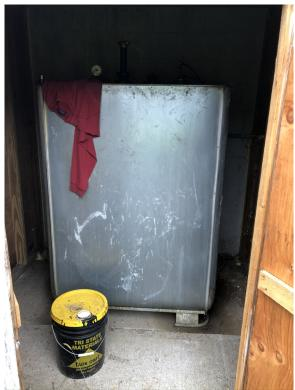
Photo 10: 275-gallon No. 2 fuel oil AST located in detached shed on the west side of the main garage.
