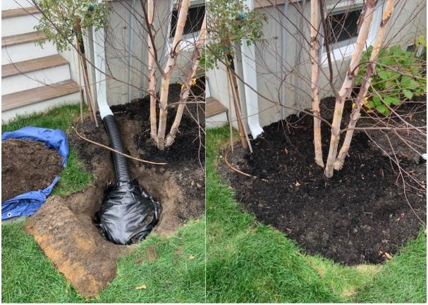
Note the filter fabric over the gravel so sand does not infiltrate the system; the peeled back sod and the under burden and topsoil collected in a tarp. Ideally, dry wells would be installed prior to landscaping but a lot of people work on the sites.
