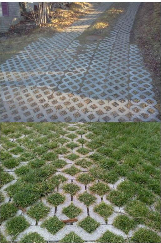
Images by Gordon Peabody. Open Faced pavers provide infiltration and habitat. We recommend these for driveways, even those on a slope.
