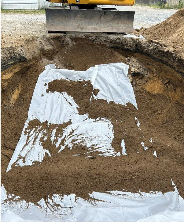
Photo 5: TP-5 demarcation placement and backfilling with clean soil
