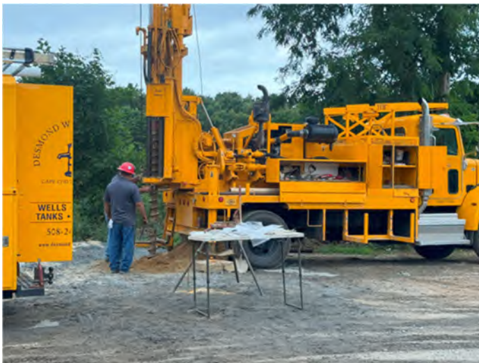
Photo 15: View of well installation in TP-5 excavation area July 29, 2024
