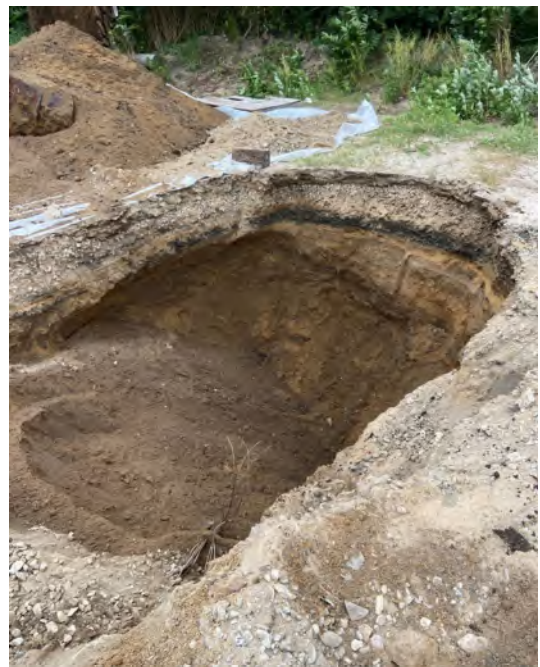
Photo 4: View of continued excavation and stockpile in TP-5
