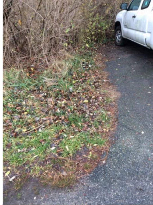
Photograph 2. Paved pullout area on the south side of Pond Road which serves as a conduit for stormwater to flow directly into the pond and wetland.
