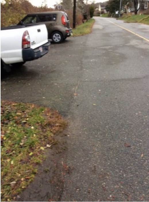
Photograph 1. Paved pullout area on the south side of Pond Road which serves as a conduit for stormwater to flow directly into the pond and wetland.
