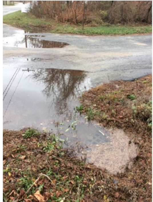
Photograph 3. Ponded stormwater and accumulated sediment at the intersection of Pond Village Avenue (on the right) and Pond Road. The ponded water nearly spans the width of Pond Village Avenue.
