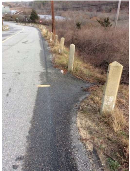
Photograph 4. The upper most paved flume on Pond Road. The vegetated area to the right likely serves to slow stormwater and promote infiltration.
