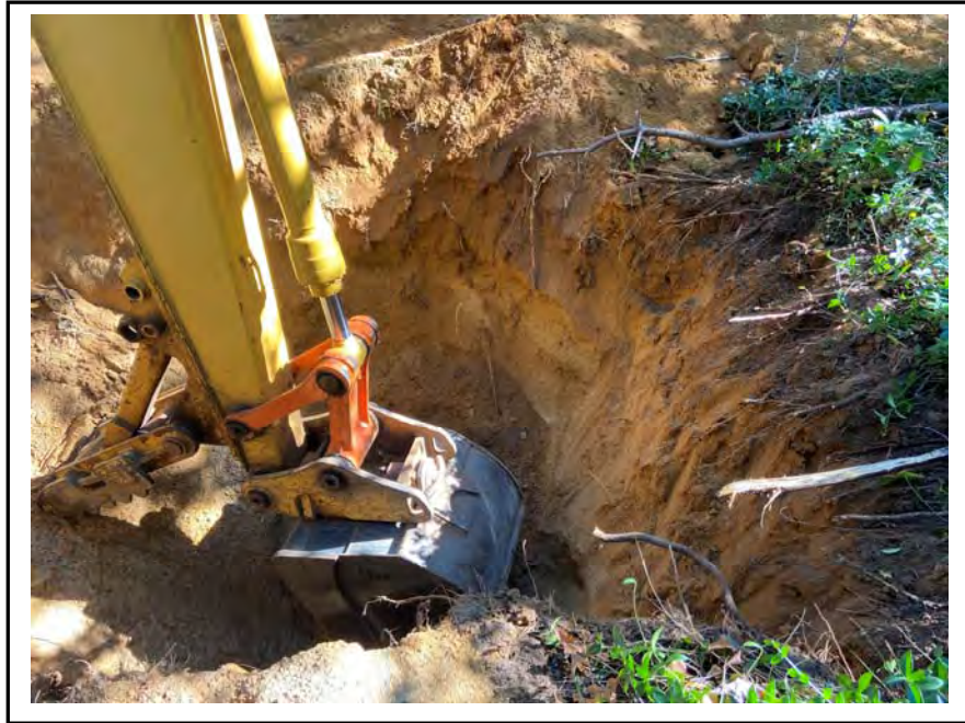
Photo 3: General test pit excavation.
