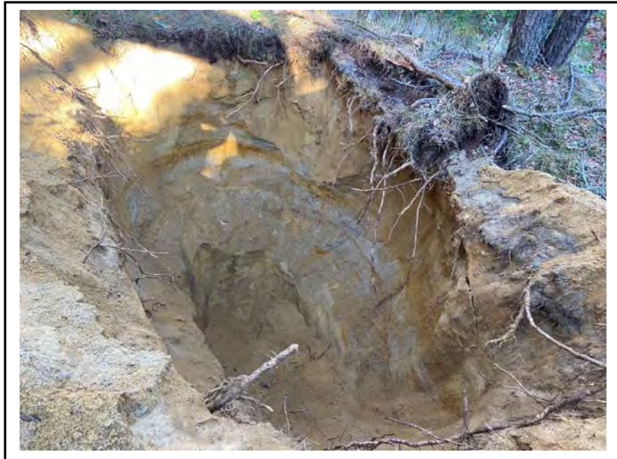
Photo 4: General test pit excavation.
