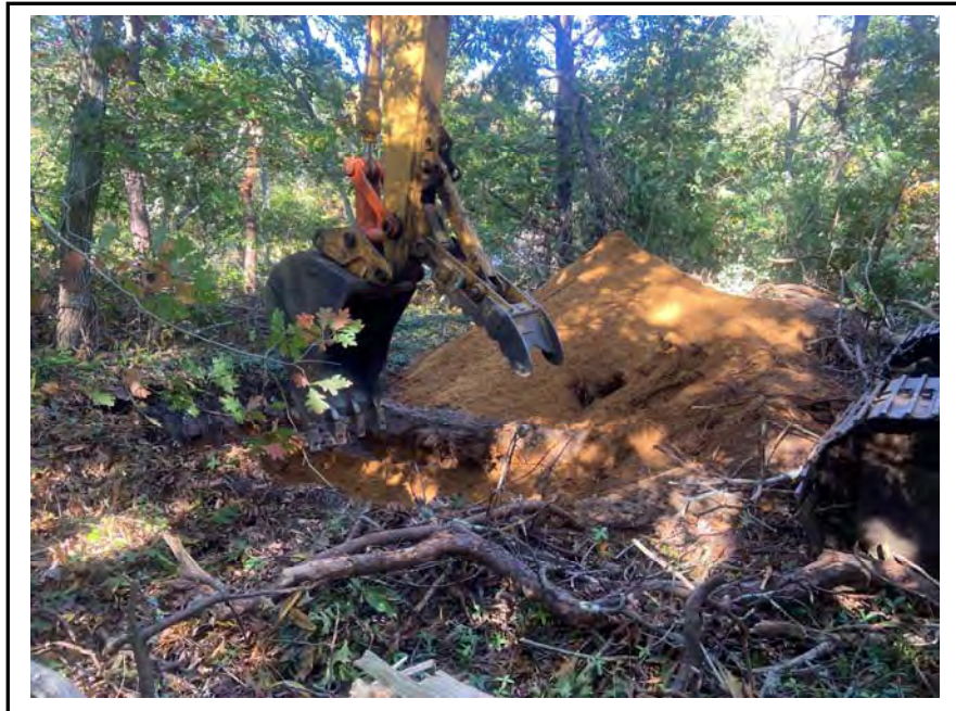
Photo 2: General test pit excavation.
