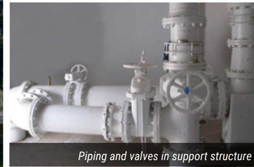
Piping and valves in support structure
