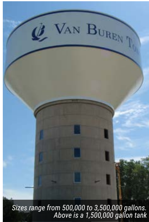
Concrete support structure requires minimum maintenance on both inside and exterior
