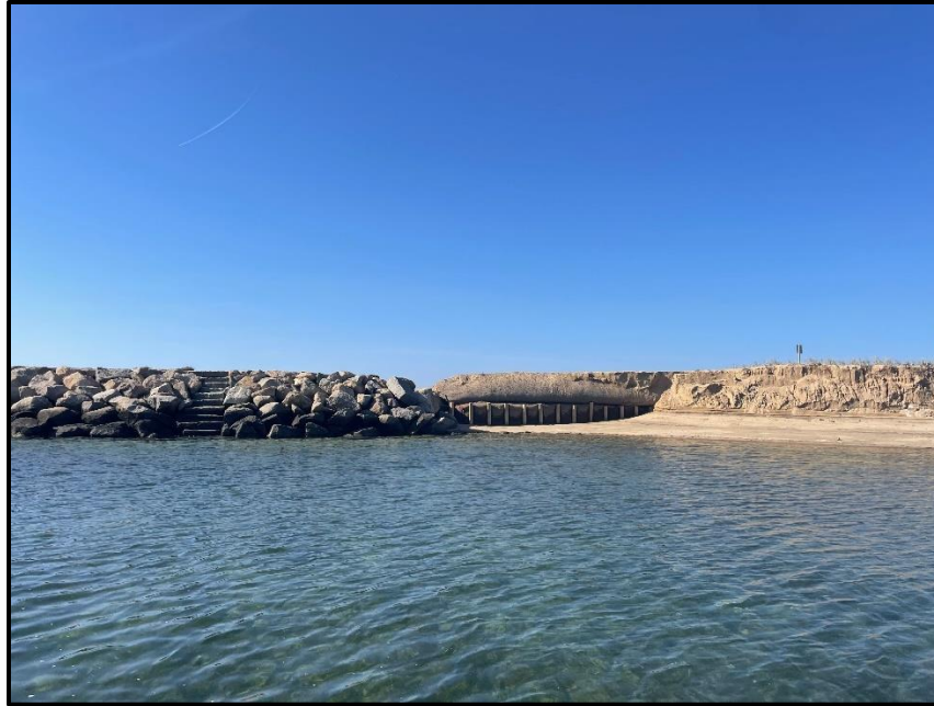
Figure 2 Photo of the bioengineered coir bag solution constructed to fill the erosional hotspot between the terminus of the north jetty spur and coastal dune (dated 10/25/2024).
