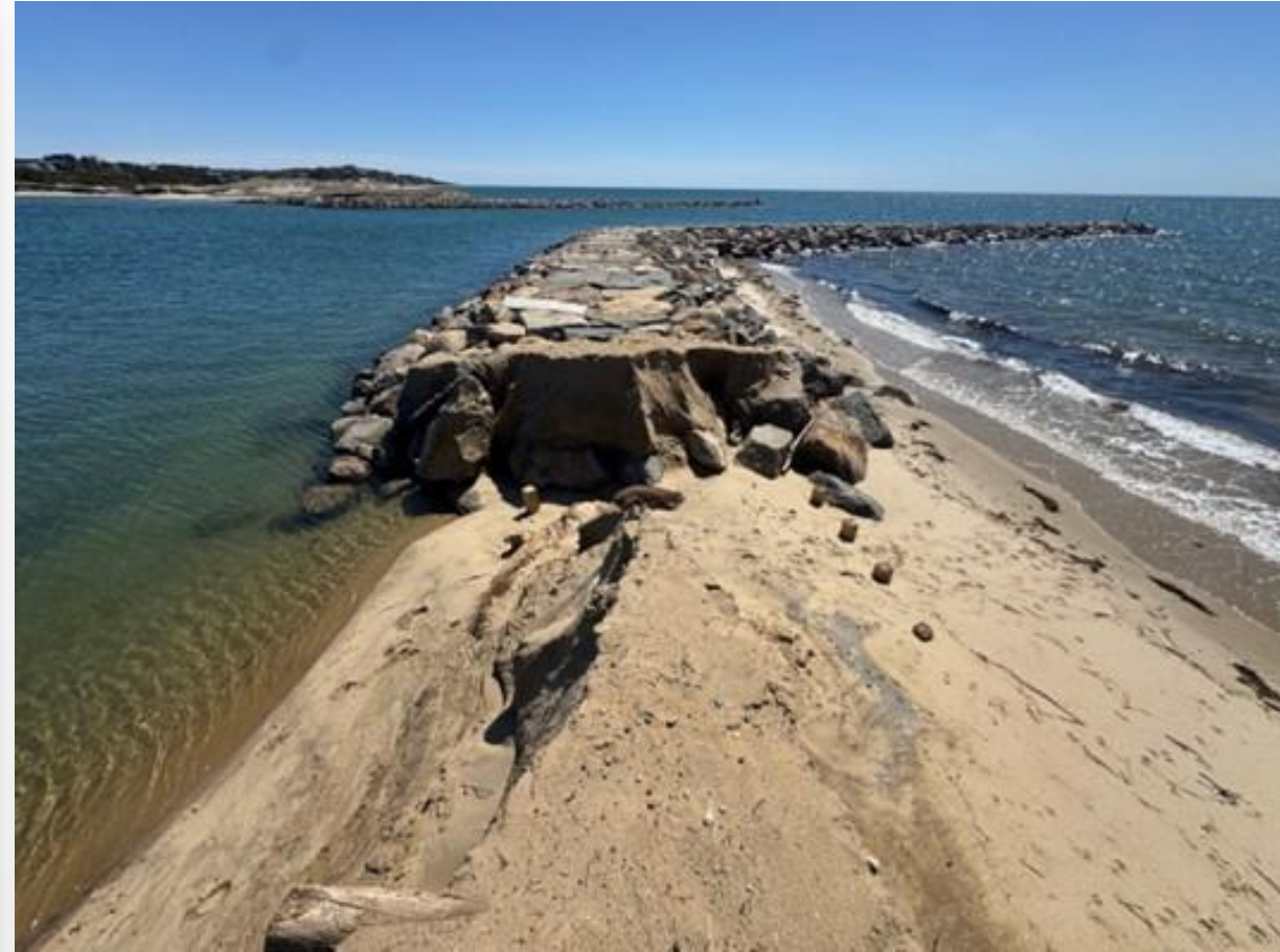
Southward view along Pamet Harbor North Jetty showing breakthrough of recently renourished area. Photo source: Environmental Partners report, 1 May 2025.
