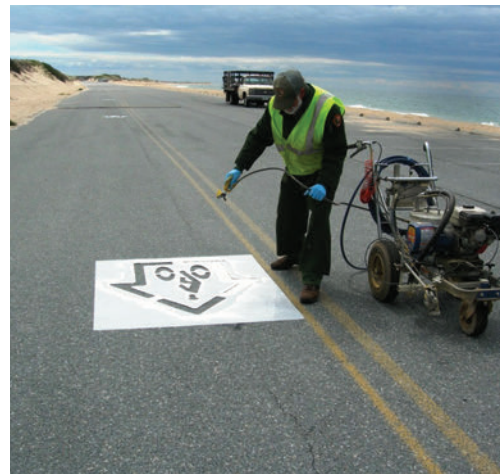
Adding a sharrow to roadway
