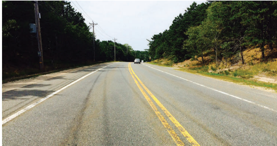
Wide shoulders along Route 6 in South Truro
