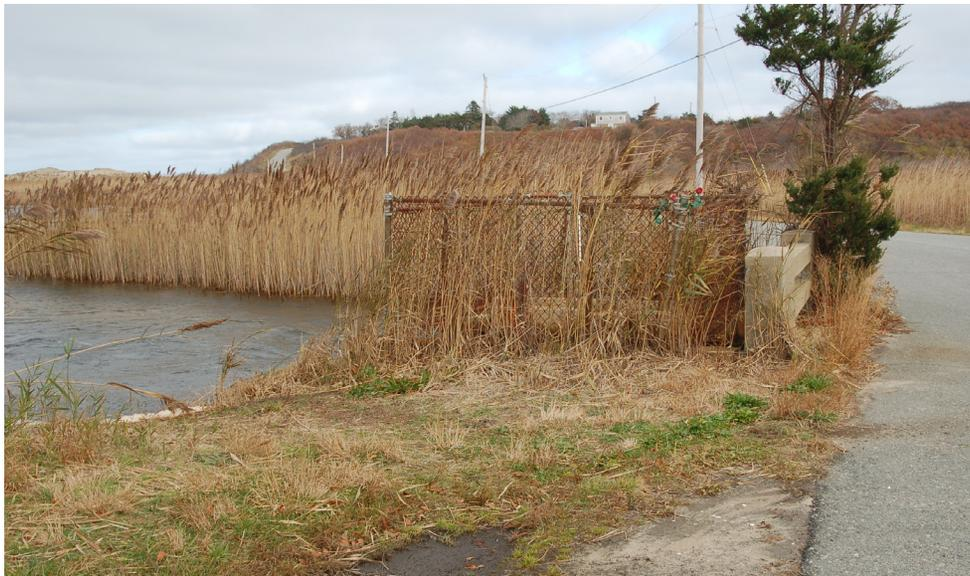
**Figure 2.2b |** High Head Road Culvert owned by the National Park Service. Built in 1956. These photographs were taken during an extreme high tide. Note that the water level is close to the road level.
